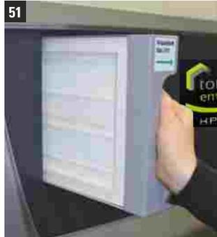
Pull the filter cassettes outwards. Replace or clean the filters by gently vacuuming them. When inserting G4 filters, ensure that the arrow points inwards. Having changed the filter, push the cassettes back
